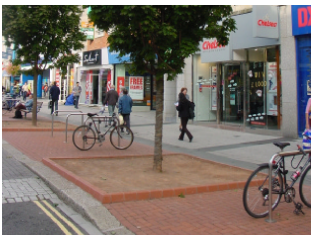
Above Bar Street - an example of bad practice - edgings to tree pits should be flush with adjoining surfaces and a contrasting colour used for the edging or gravel to warn visually impaired people of a change in surface finish
