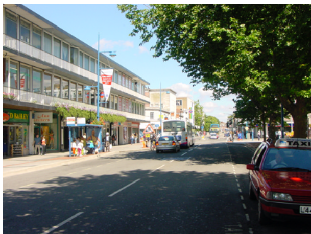
Above Bar - Refurbishment of the whole street and placement of street furniture in zones provides better pedestrian access
