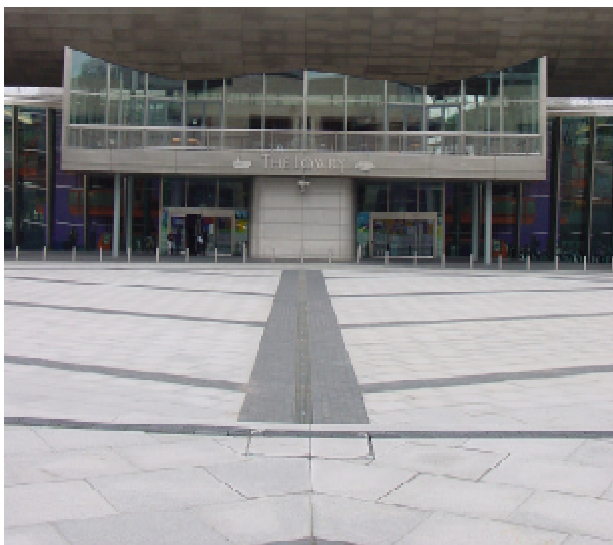
Salford - Paving at the Lowry Centre
