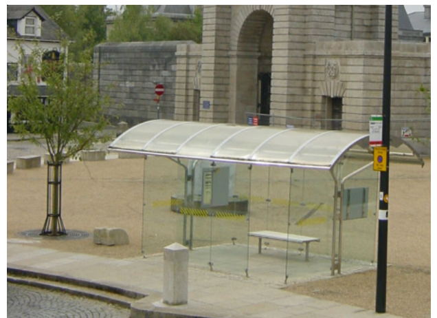
Stainless steel bus shelter with granite bollard, Plymouth (N.B Kerb details are not in accordance with SCC accessibility standards)
