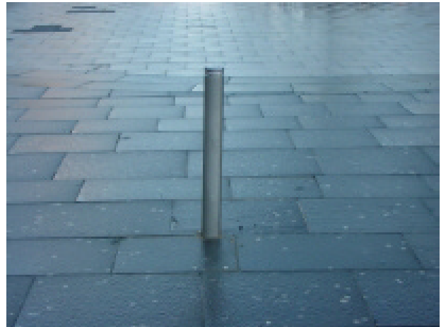
Existing stainless steel bollards, in the Above Bar precinct, are too short and are not visible to people with visual disabilities
