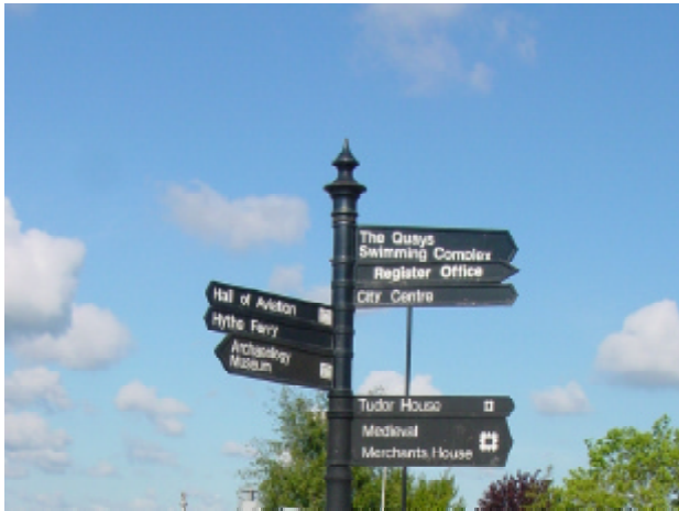
Cast iron painted finger posts are easily vandalised, but the white lettering on a black background is legible to the partially sighted
