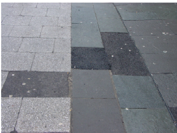
Adequate supplies of paving should be available so that replacement with black top is not necessary
