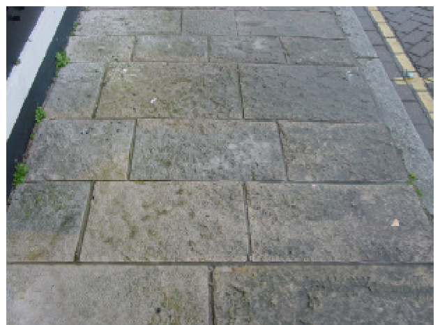
Purbeck natural stone paving slabs with a scabbled finish, Cement Terrace
