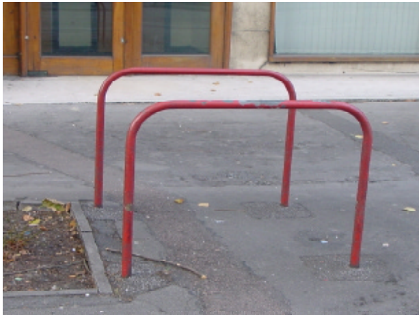
Bicycle railings suffer from heavy use so painted finishes deteriorate quickly
