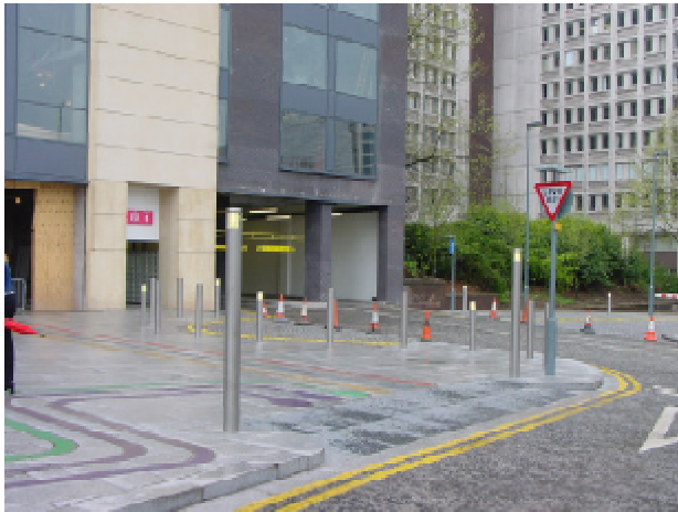
Silver grey painted lighting columns and bollards, Birmingham give a coordinate appearance, however illuminated bollards can conflict with the use of CCTV and frequently targetted by vandals
