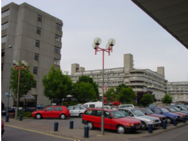
North Western character area - the Central Station concourse needs to be enhanced to reflect its importance as a key arrival point
